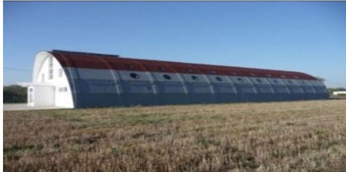
Fig. 1. Prefabricated hall made from ferrocement sandwich elements
